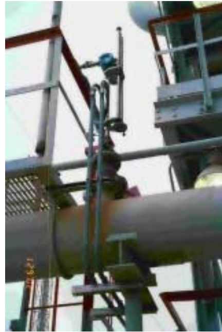
Figure 1: 454FT with Retractor/Restraint in 16" Line
