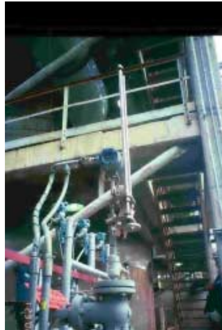
Figure 2: 454FT with Retractor and Customer supplied valve.
